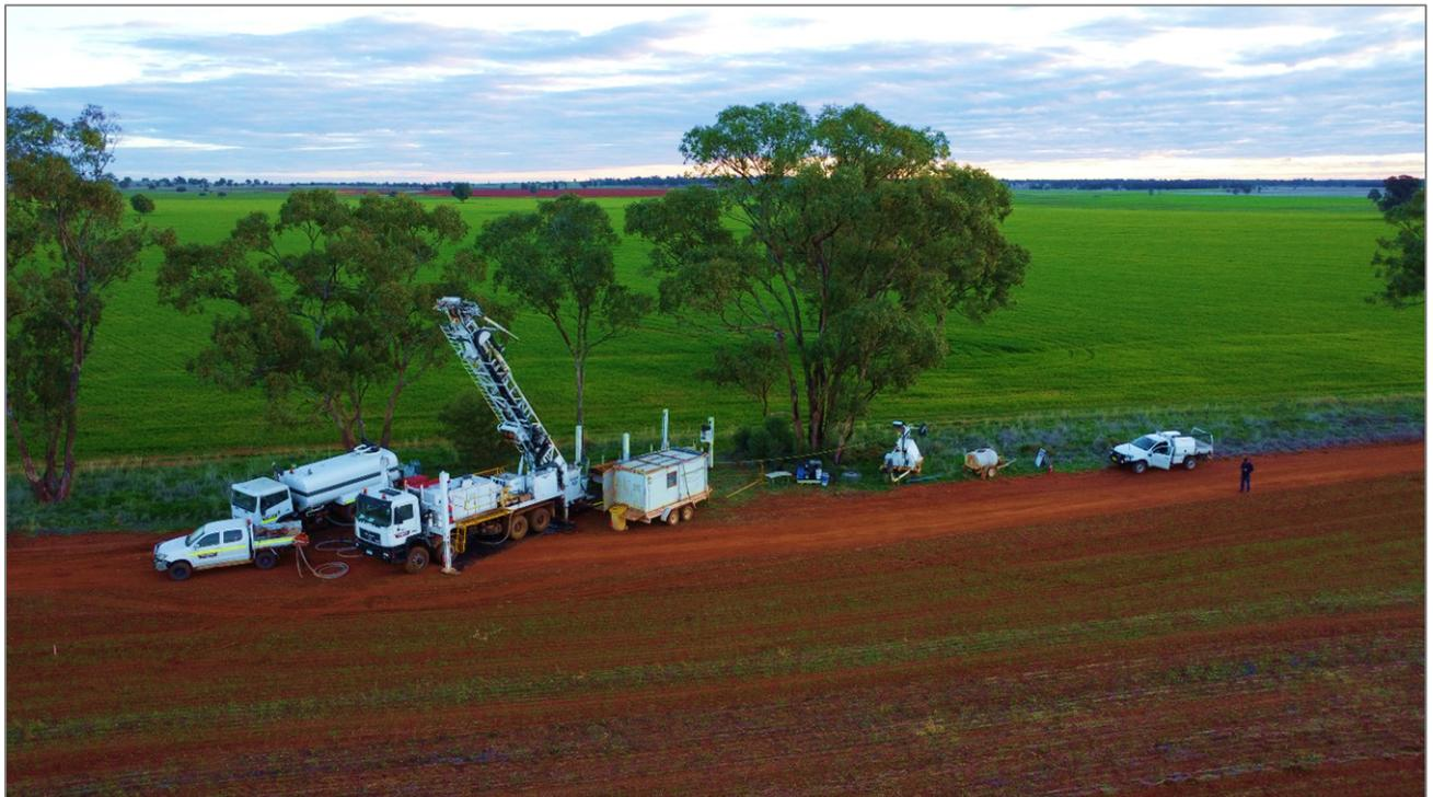
**Figure 1: Diamond drilling operations underway at the Melrose prospect. Note the drill rig has been positioned along a fence to avoid damage to fresh crops.**
