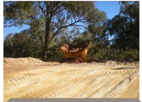
*New ramp established to house a 40t hopper addition to the processing circuit*
