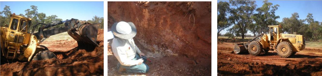
Excavation works commenced on Pit One and MC306, with gravel layers mined, stockpiled and processing underway. The bedrock is now revealed in parts. 15m x 50m sections are planned using trenches as orientation tools for depth to gravel and bedrock.
