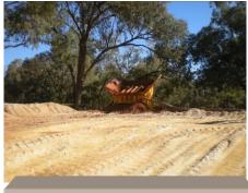
New ramp established to house a 40t hopper addition to the processing circuit
