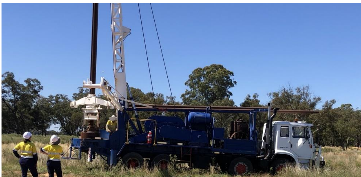
Figure 3: Platina Lead Drilling
